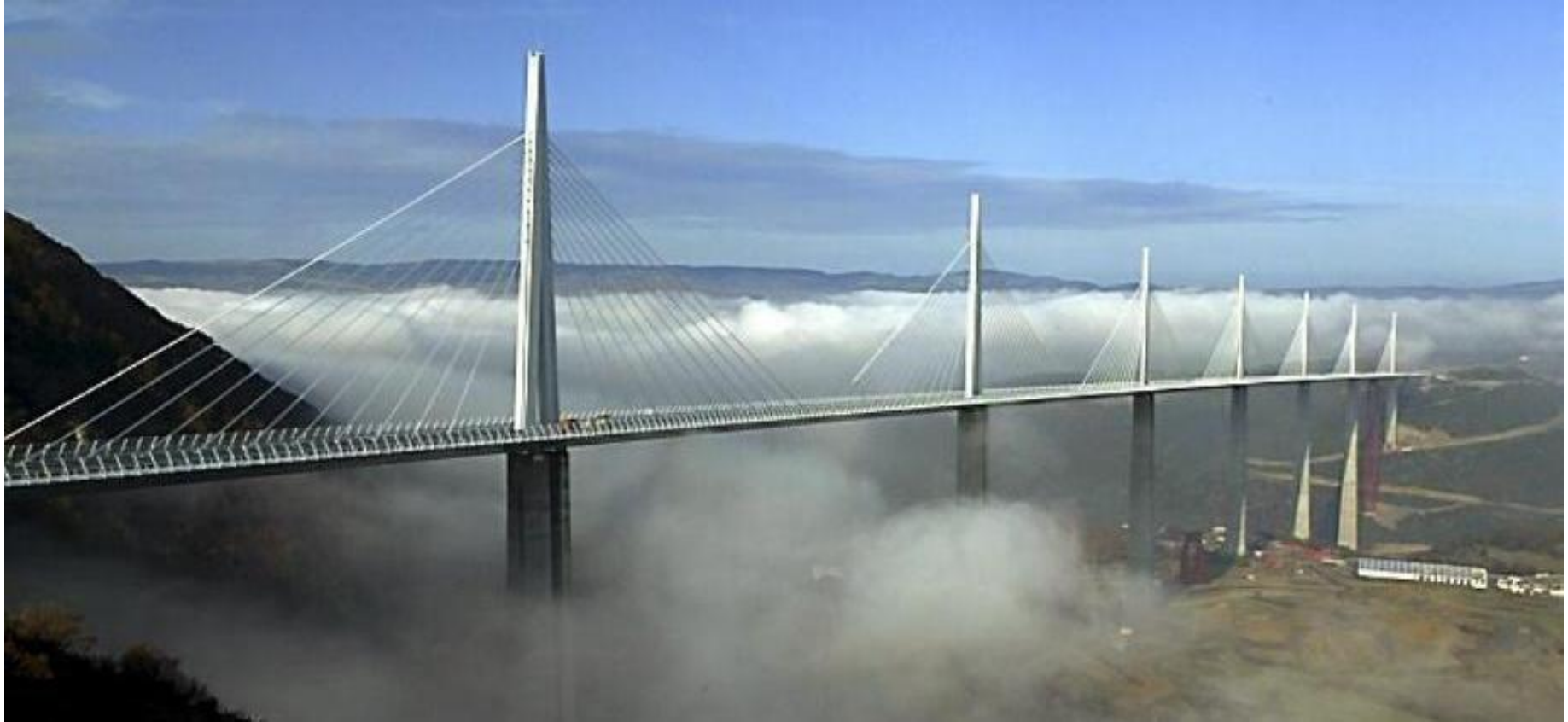
Millau Viaduct, France. 2004, designed by Sir Norman Foster Tallest bridge in the World
